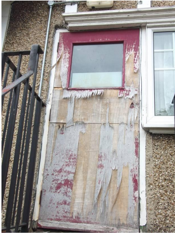
Photograph 19 (Second floor fire exit door)
