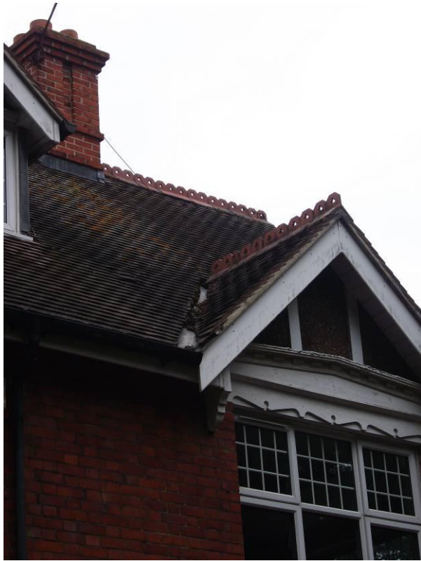
Photograph 03 (East elevation roof)
