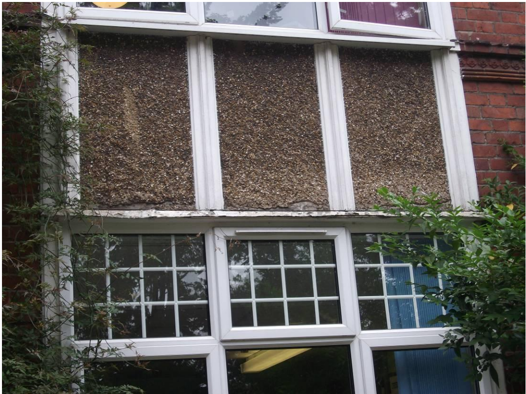
Photograph 04 (East elevation render infill)
