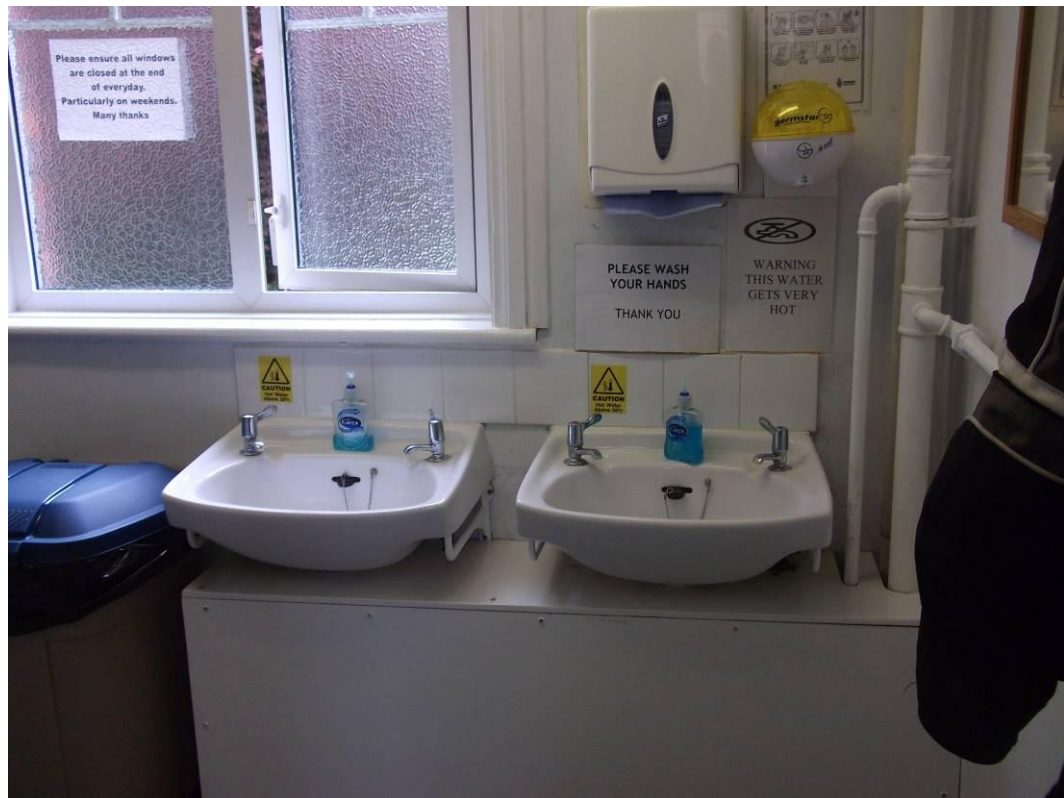
Photograph 14 (first floor toilets)
