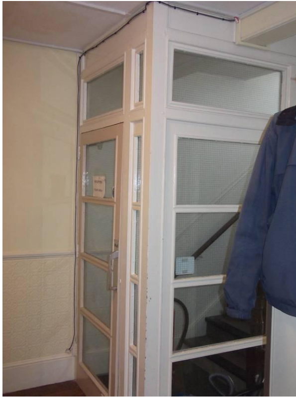
Photograph 13 (Fire door to stairs first floor)
