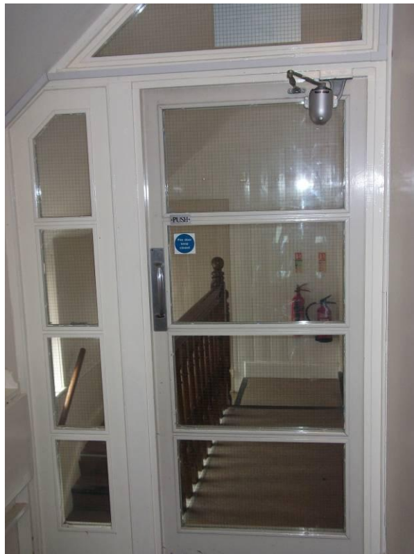
Photograph 10 (Fire door second floor)
